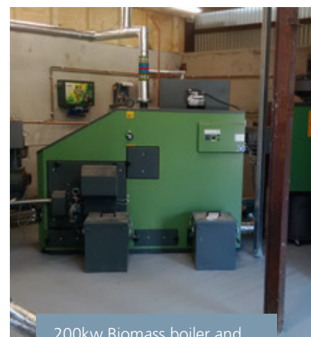
200kw Biomass boiler and district heating main provides all heating and hot water for eight properties on and close to the farm. Fuel for the boiler is collected waste wood from the local saw mill and sustainable tree thinnings
